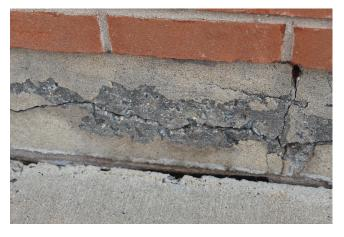
Based on my evaluation and assessment, nothing I observed or evaluated would enable me to assign a CFSIC-related severity class coding. In the absence of definitive map cracking, efflorescence and staining it would be prudent to schedule the extraction of core samples for petrographic analysis because of the building's use as a public structure. Although we believe the cause of the suspicious cracking and spalling is associated with the application of
