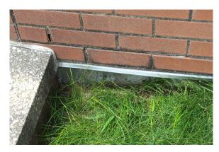
At first glance the horizontal cracking and surface spalling could resemble the appearance of pyrrhotite laden concrete from that period, yet the damaged area was isolated to the short section of the wall in contact with the sidewalk, an area exposed to constant deicing chemicals over the past 14 years. The remainder of the three-sided addition showed no signs of concrete surface defects outside the normal hardened shrinkage cracks which were very small and infrequent.
